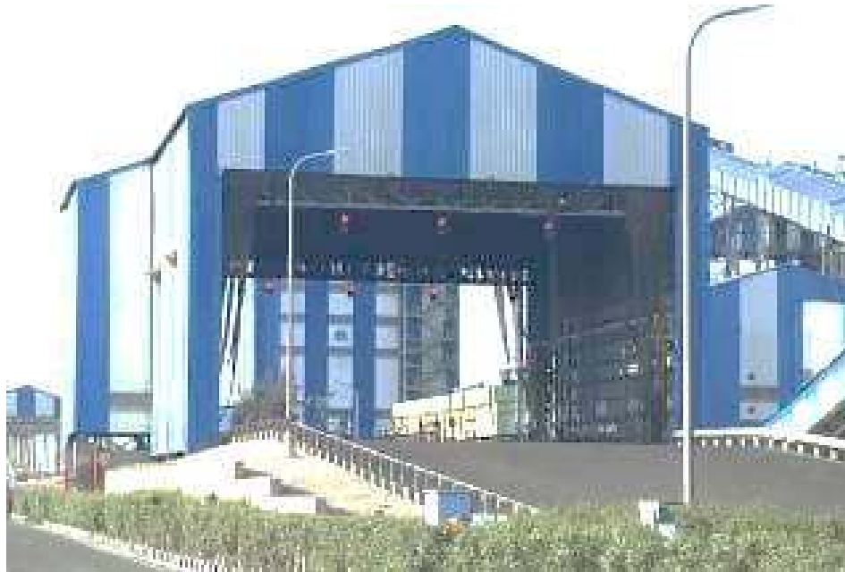
Coal Unloading Bay
