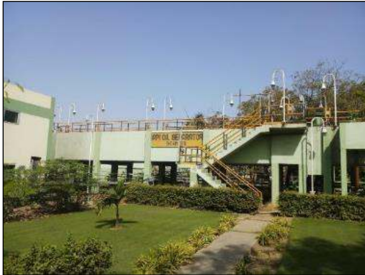
Oil Separator Unit
