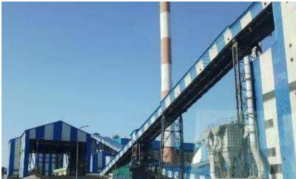
Covered Conveyor Belts
