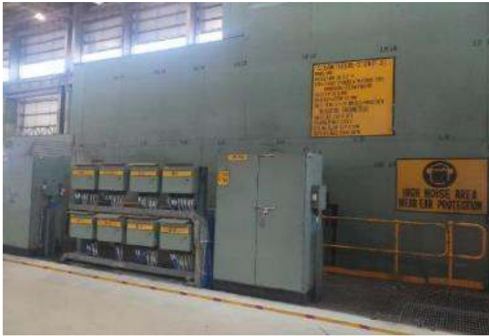
Acoustic Enclosure for Turbines
