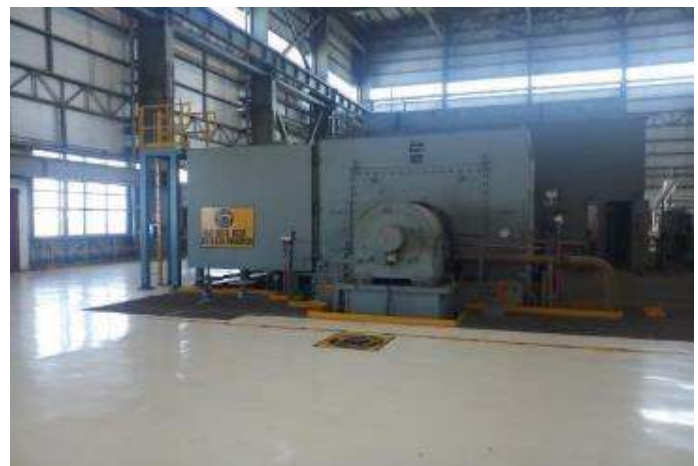
Acoustic Enclosure for Generators
