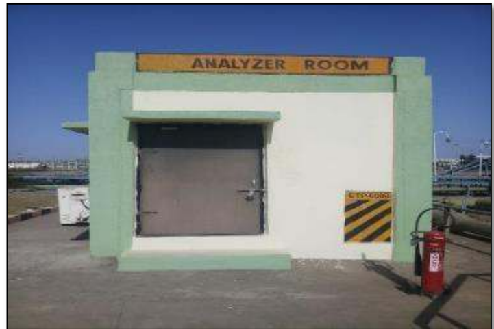
Analyzer room for Continuous Effluent Monitoring System
