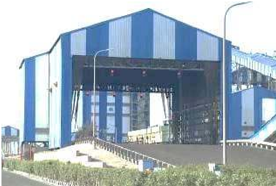
Coal Unloading Bay
