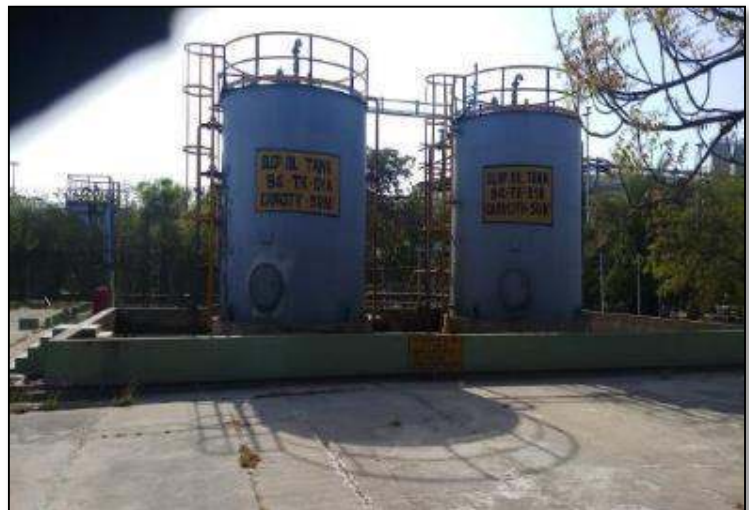
Slop Oil Storage Tanks
