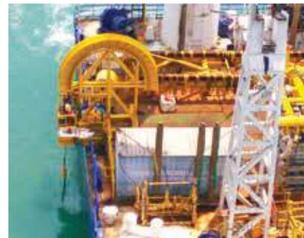
Umbilical Installation at Live Platform (CRP)
