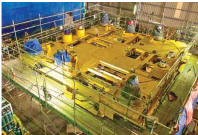
Fabrication of Subsea Structure
