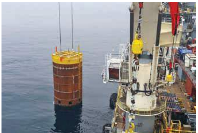
Subsea Structure Foundation Installation
