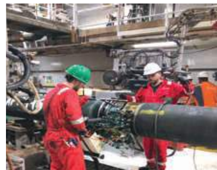
Deepwater Pipeline Installation Pipes being welded at welding stations
