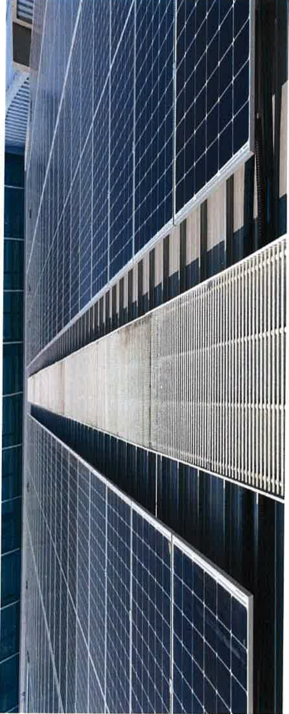
Installation of Solar Panel outside the PMD Site
