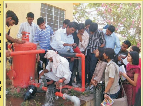
Er. J K Gaur explaining filter system to B Sc Ag (Plasticulture) students
