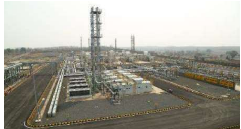
Installation of GGS-11 completed
