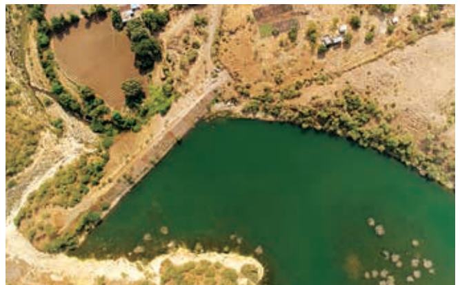
Water conservation through earthen dam construction
